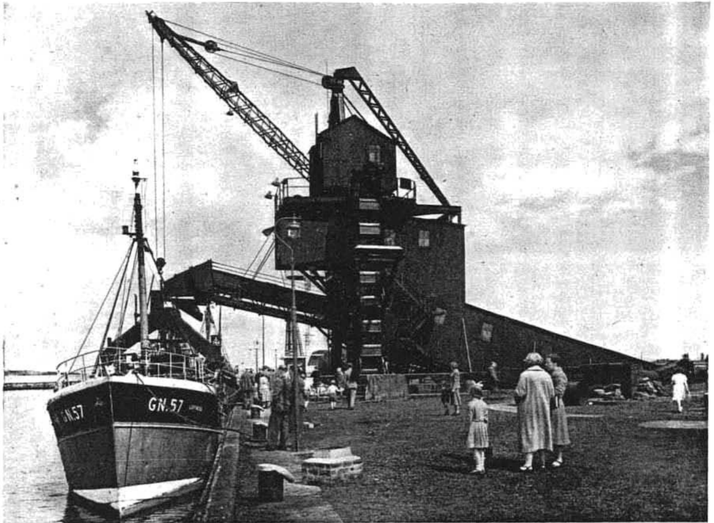
BUNKERING A TRAWLER AT THE COAL CONVEYOR, MIDDLE PIER
