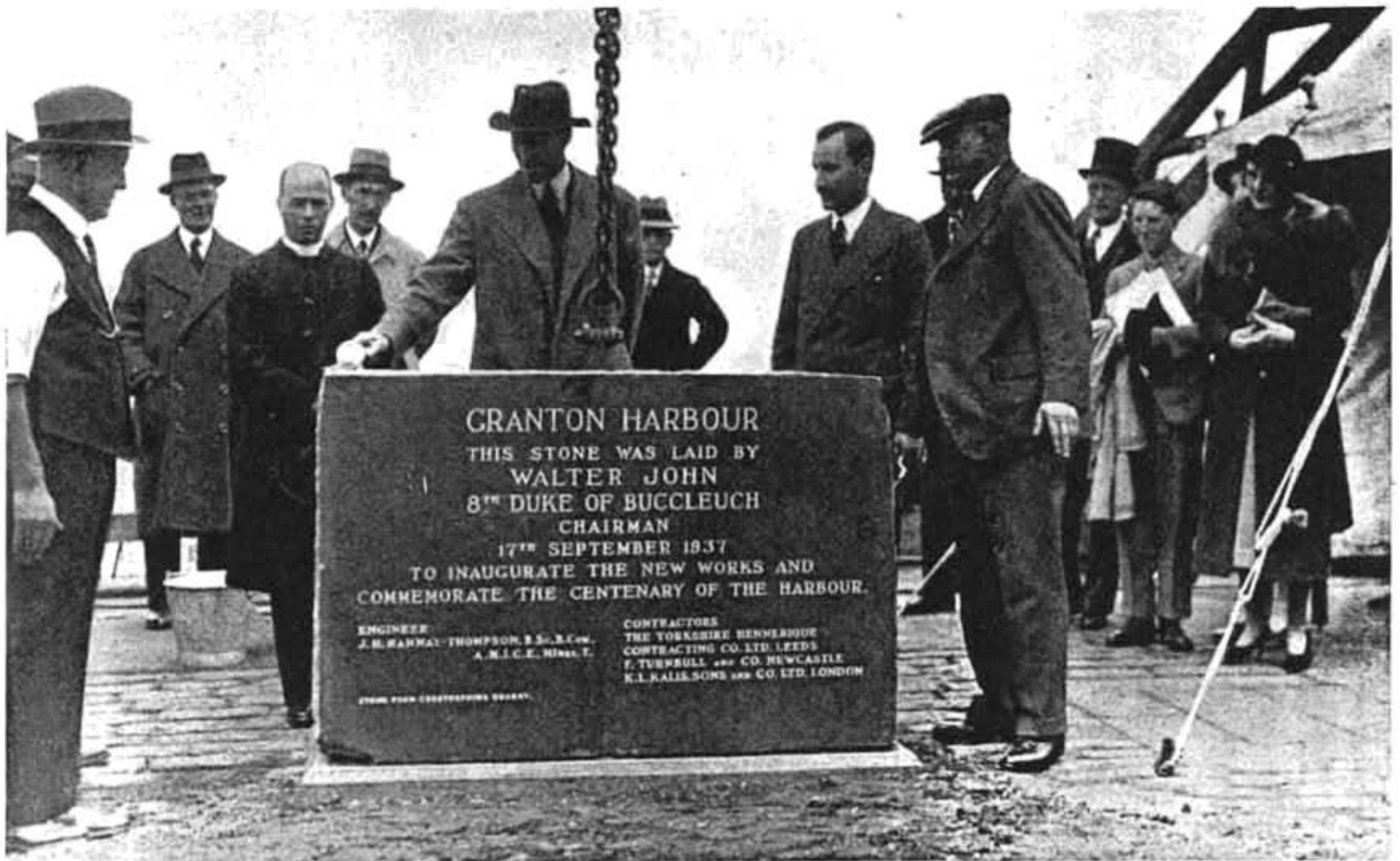
THE CHAIRMAN LAYING THE FOUNDATION STONE OF THE NEW COAL JETTY AT MIDDLE PIER, SEPTEMBER 1937
