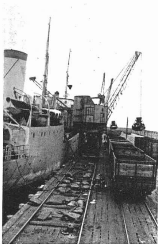
DISCHARGING TIMBER (left), AND DISCHARGING COAL BY GRABS AT WEST PIER
